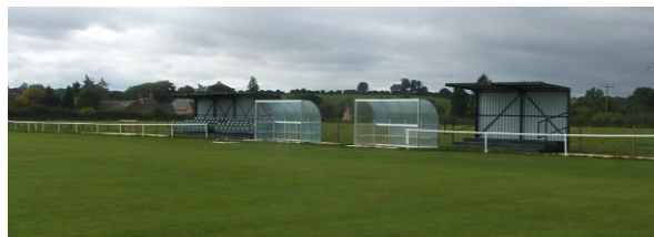
New covered spectator accommodation and dug-outs
